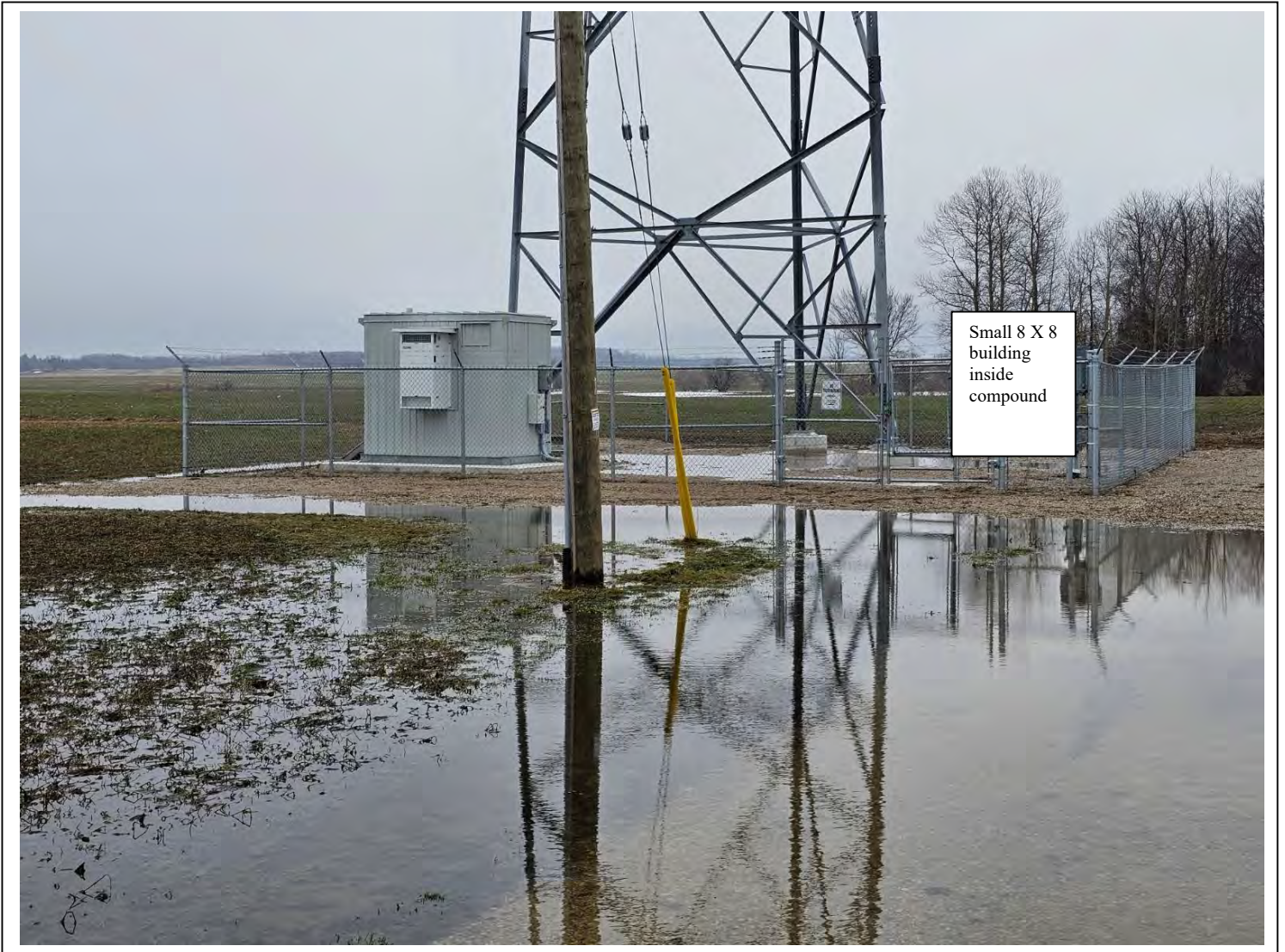
Small 8X8 steel clad building inside compound for fire and other services
