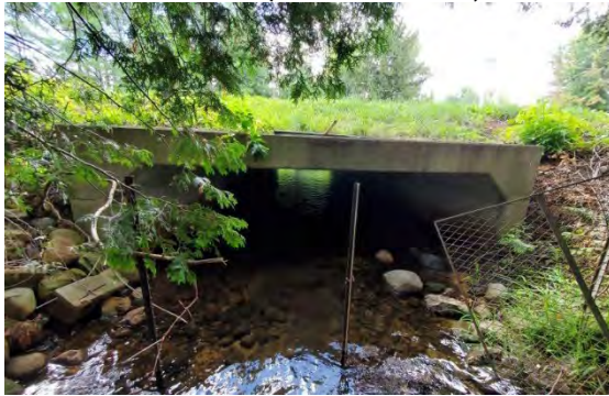
Gorrie Line Rectangular Culvert (BCI=21 Poor)
