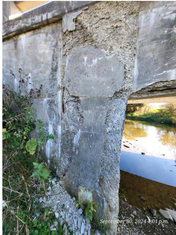
09 - NE Wingwall Delamination
