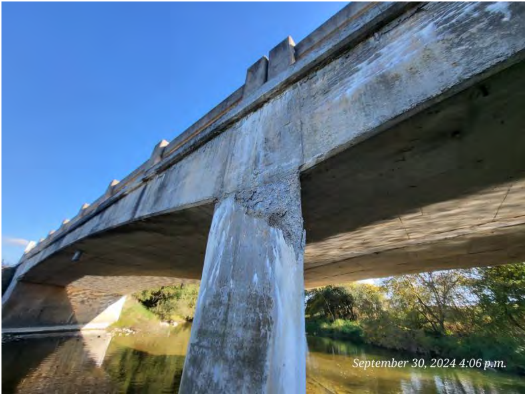
11 - North Pier Spalling
