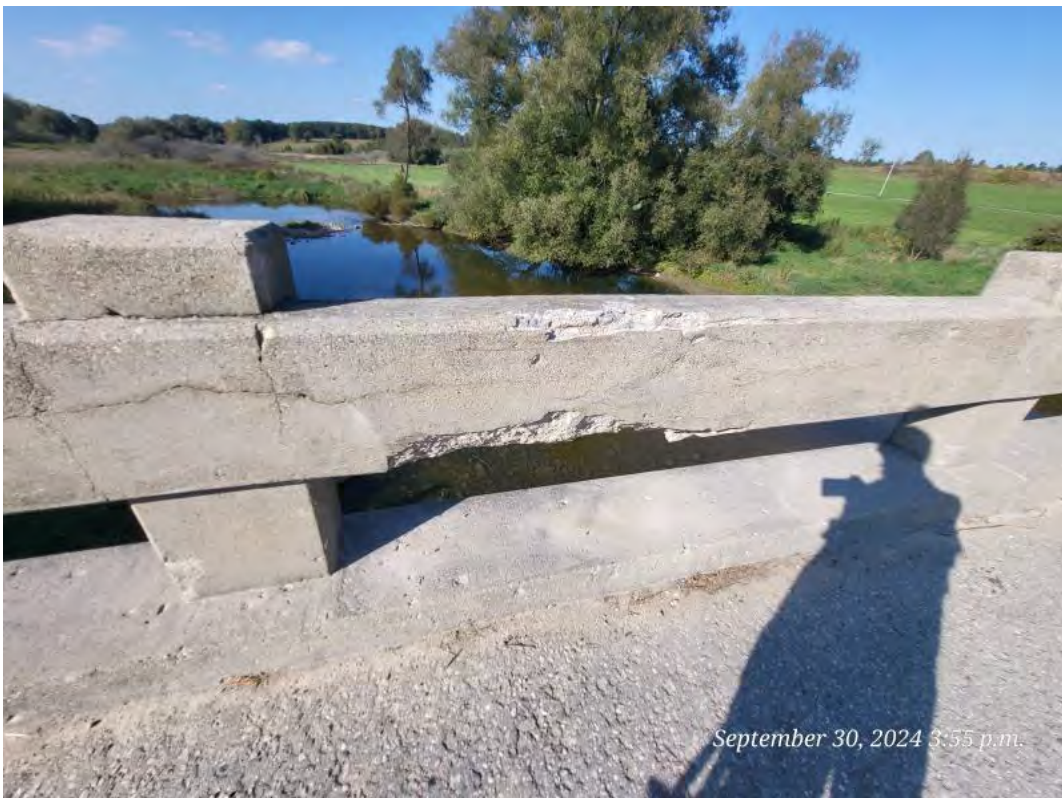
12 - North Railing Spalling
