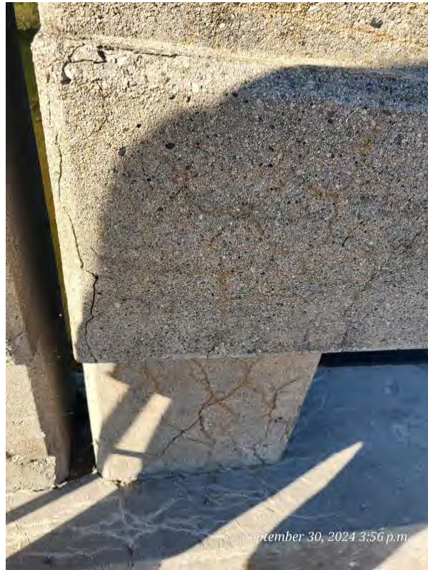
15 - Railing Cracking
