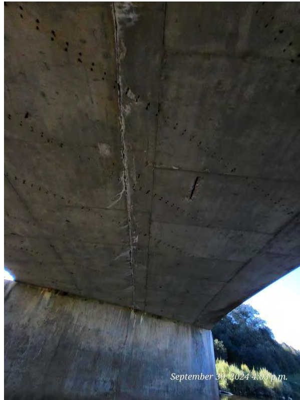
07 - East Span Deck Effloresnce
