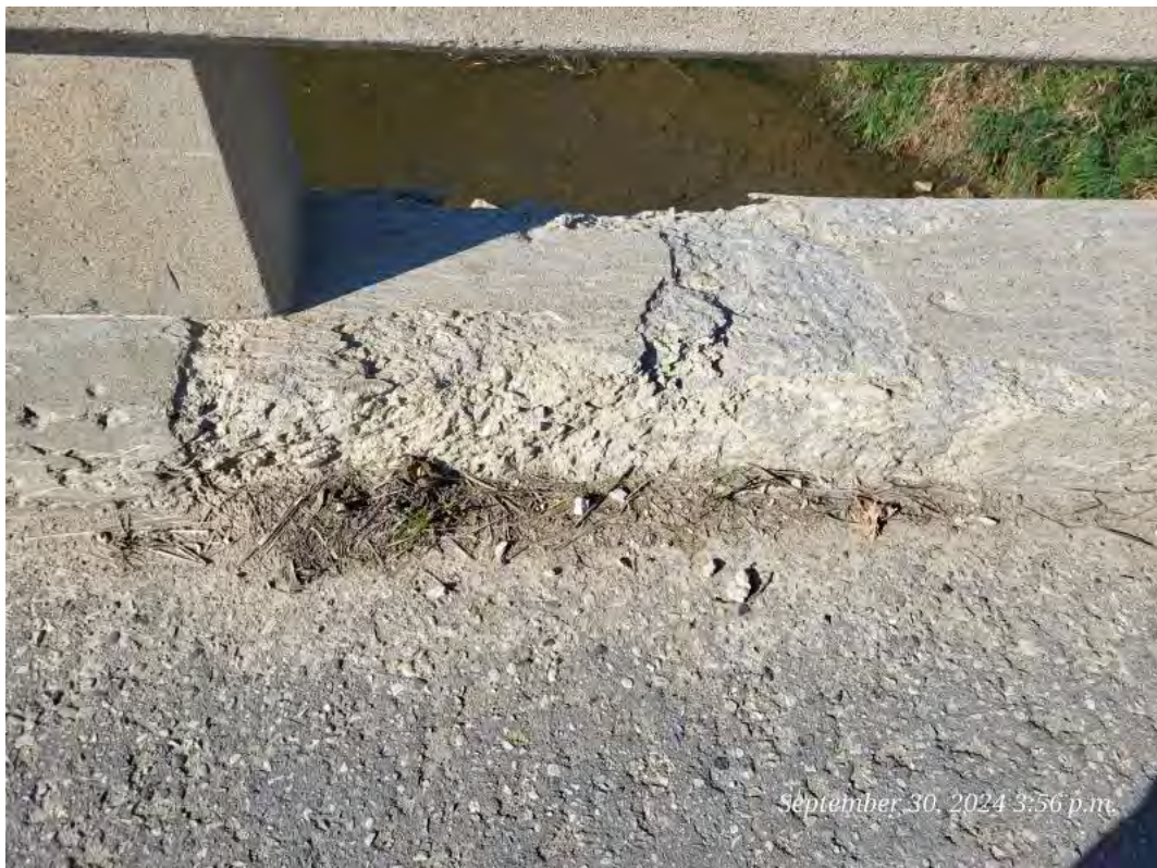
10 - North Curb Spalling
