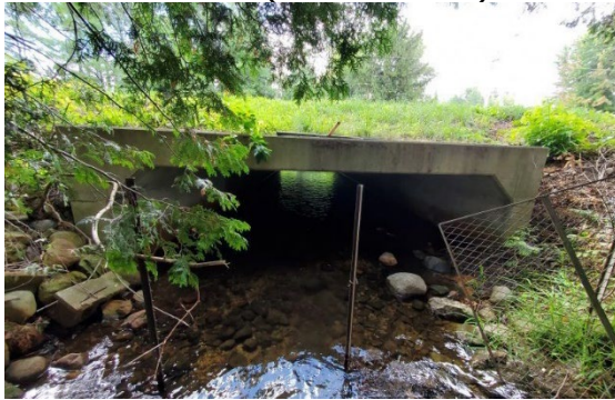
Gorrie Line Rectangular Culvert (BCI=21 Poor)
